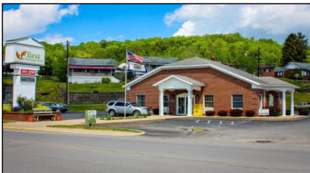
Fairview Office 309 Main Street Fairview, WV 26570 Phone (304) 449-1700 Fax (304) 449-1967
